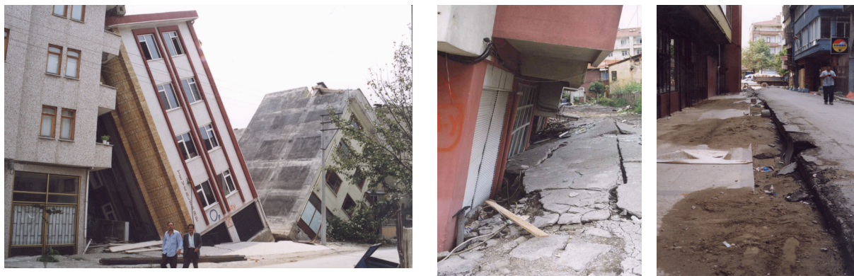
Figure 1. Examples of bearing capacity failures of shallow foundations in Adapazari
