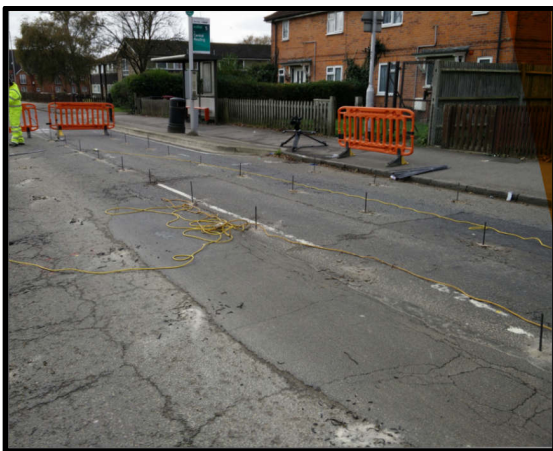
Figure 1: Northumberland Avenue - Reading, UK; location of the treatment and of the Ground Penetrating Radar Survey.
